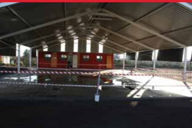
Designated areas for MMC appointments, repeat visits and HIV Counselling and Testing
