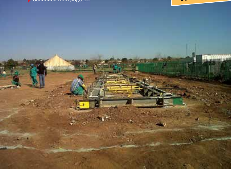
Construction crews hard at work . . .
